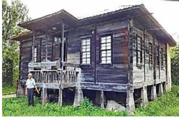
Figure 7. A historic house constructed with high subbasement against floods in the Samsun - Çarşamba floodplain.
